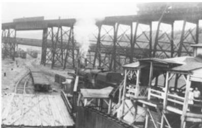
Extensive work on the Genesee docks made use of a multiplatform trestle to use gravity to transfer coal from bins into cars to go into the holds of the vessels.
